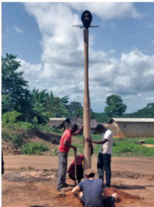
LiFi LED technicians set a solar power LED LiFi technology-enabling pole.
