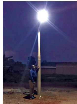
Ange Frederick Balma is standing at the base of this solar powered LED LiFi transmission pole in Africa.
